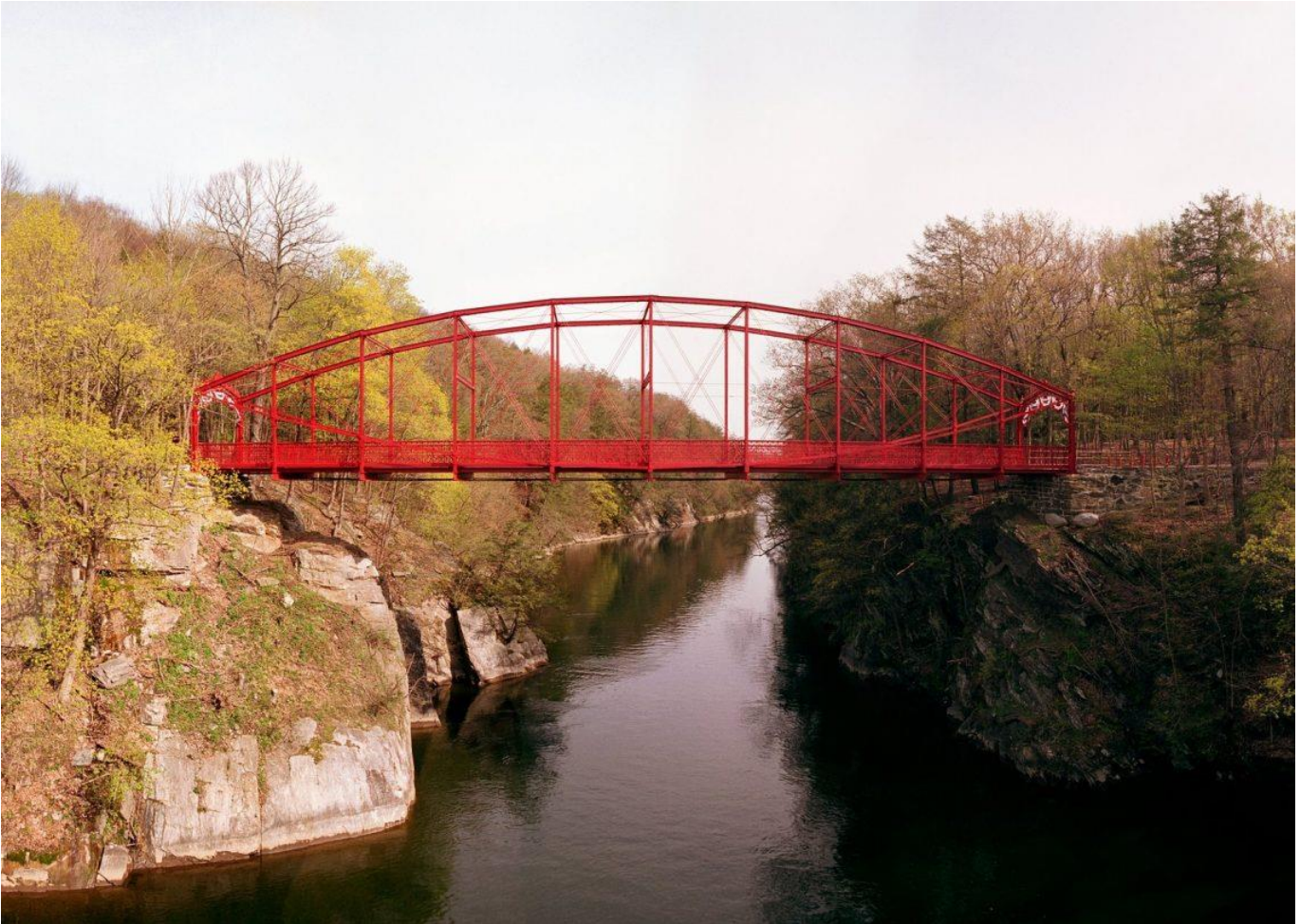
The 1895 iron bridge at Lover's Leap, New Milford, photo by Timothy Stobierski
